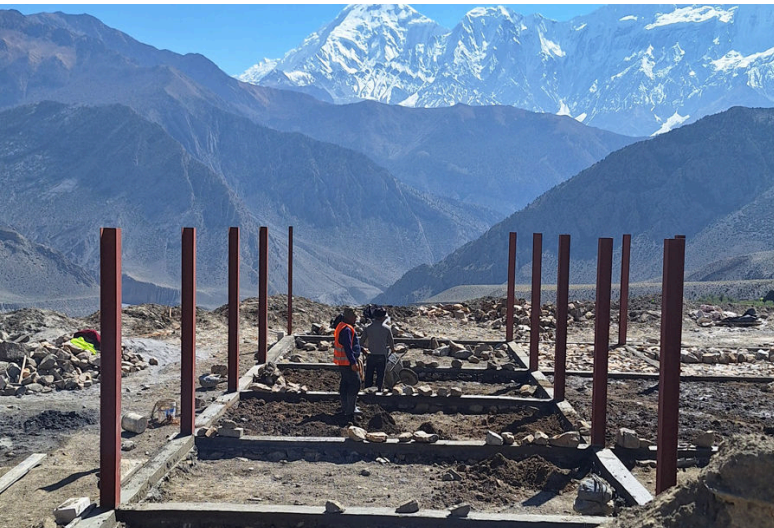
Early October: strip foundations and H-profile posts are set.
