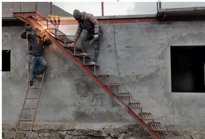
Below: The external staircase leading to the roof being welded
